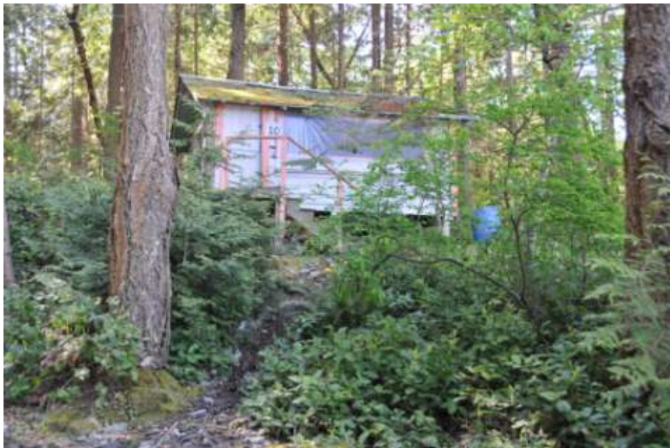
Figure 16. Relatively undisturbed forest around some cabins included in Conservation zone
